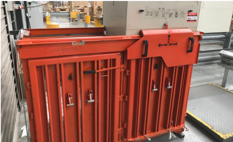
Baler installed at L'Oréal's Melbourne production facility compacts label liner waste into large 500kg bales
