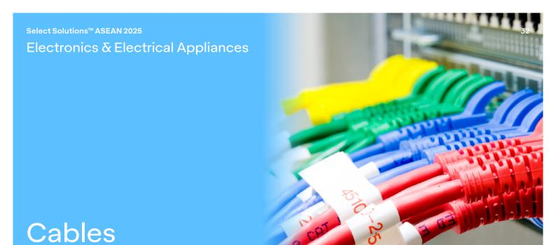
Keeping track of cables in cabinets, workstations and offices is essential when installing, repairing or troubleshooting. Reliable part identification and branding depend on good printability, usually with thermal transfer printers and ribbons. Smaller diameter cables need more flexible films and higher performance adhesives. Avery Dennison Cables portfolio
